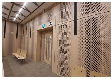
Perforated Acoustic Panels is a kind of acoustic product that has holes on both sides high density board. Various panel sizes and hole diameters are available for your selection.
